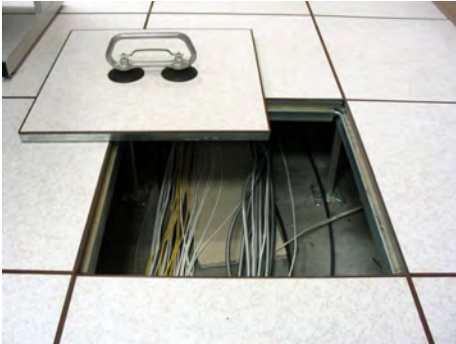
The typical under-floor access.
