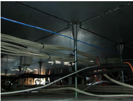
The typical under-floor condition.
